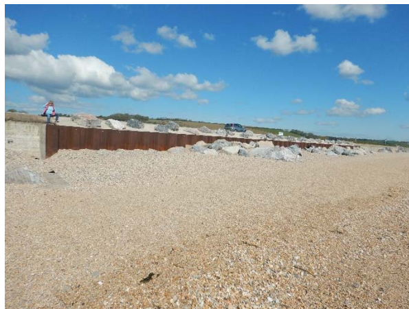
Figure 3-10 Repaired ~60m section of concrete seawall, showing sheet piles, rock/concrete crest protection and rock armour at the toe
