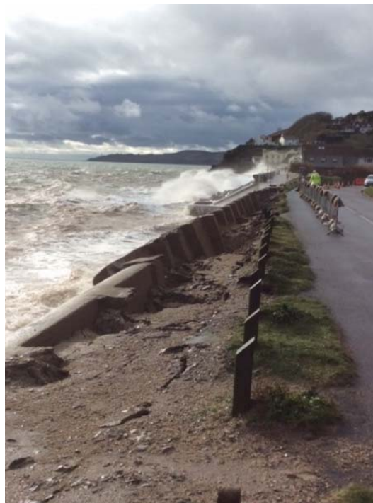
Figure 3-9 Collapse of a section of the concrete seawall running north of Torcross in February 2016
