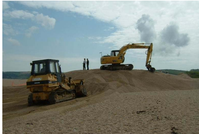
Figure 3-7 Beach material being redistributed over bastion
