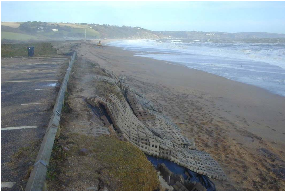
Figure 3-2 2001 Storm damaged 'armour flex' blockwork protection
