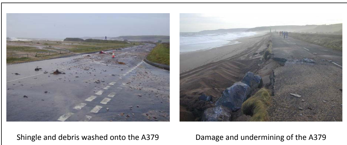
Figure 3-3 2001 storm damage to the A379
