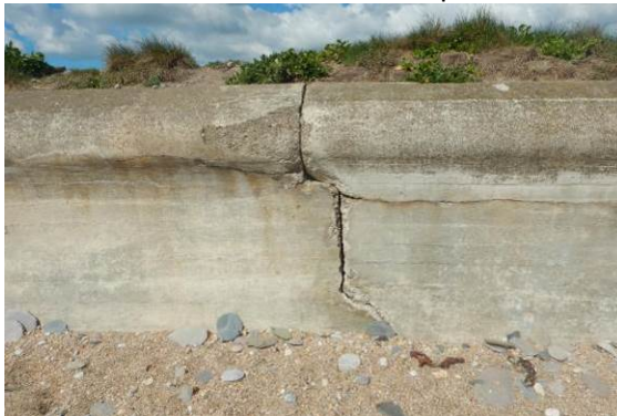
Typical vertical crack found at joints in wall
