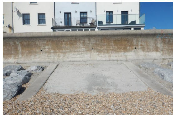
Concrete revetment with no rocks
