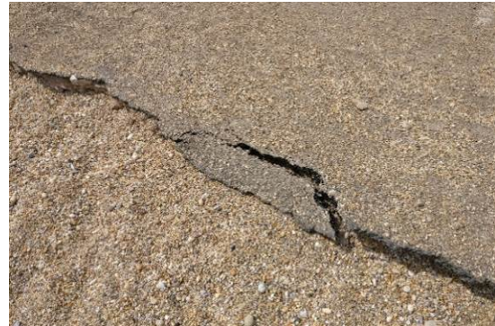
Cracking of tarmac within the car park due to undermining
