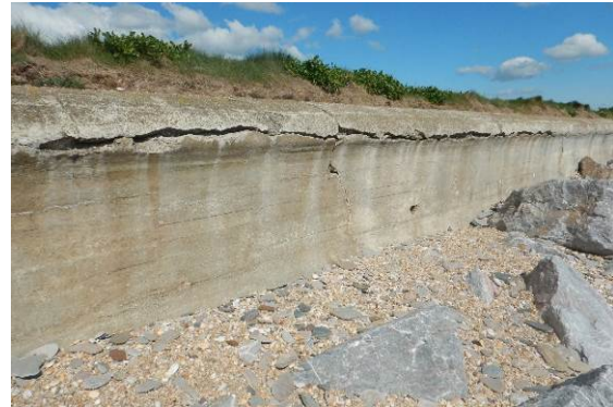
Major horizontal crack along top of the wall
