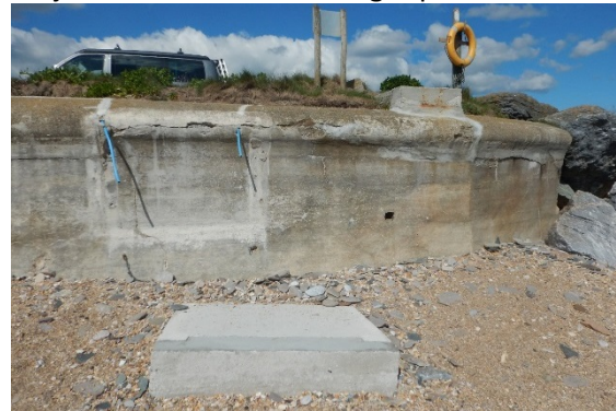
Evidence of patch repairs to northern end of wall
