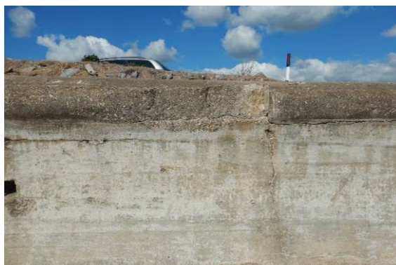
Evidence of concrete cracking
