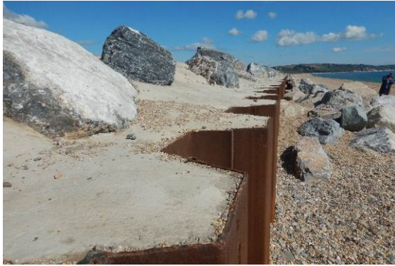
Sheet pile with concrete back fill
