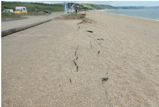
Cracking of the carpark as result of erosion
