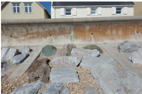
Green paint indicating the location of patch repairs
