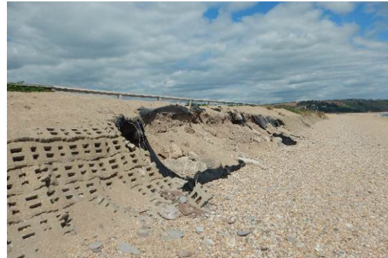
Large area exposed due to washout of blocks
