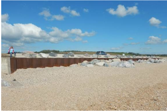
Sheet pile wall north of the slipway
