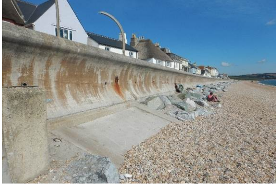
Concrete recurve wall with sloped revetment providing a flood defence to properties at Torcross
