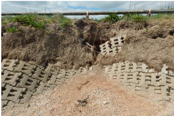
Slumping of the defence with nylon cords visible
