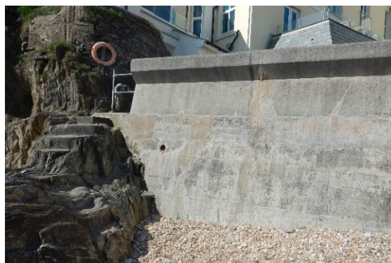
Southern end embedded into bedrock/cliff
