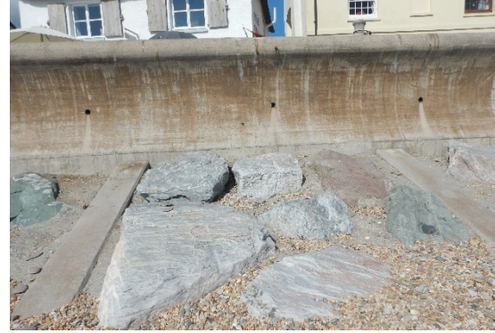
Typical section of wall showing rocks embedded in the revetment
