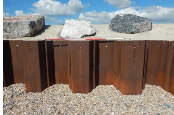
Sheet pile with 2m ranging pole for scale
