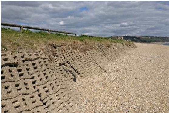
‘Armourflex’ blockwork
