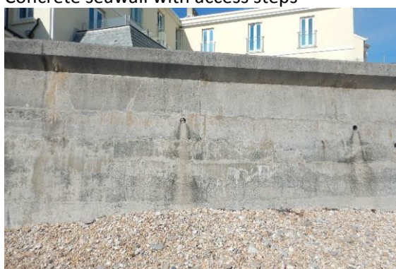
Middle section showing rust staining and surface cracking
