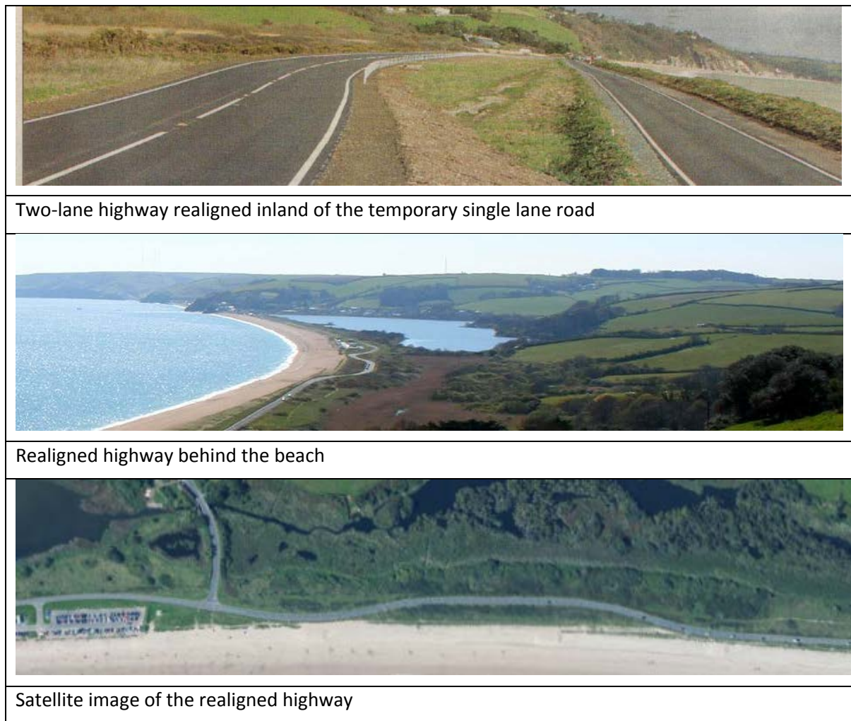
Figure 2.3 New section of road set back 21m from the existing storm damaged section
