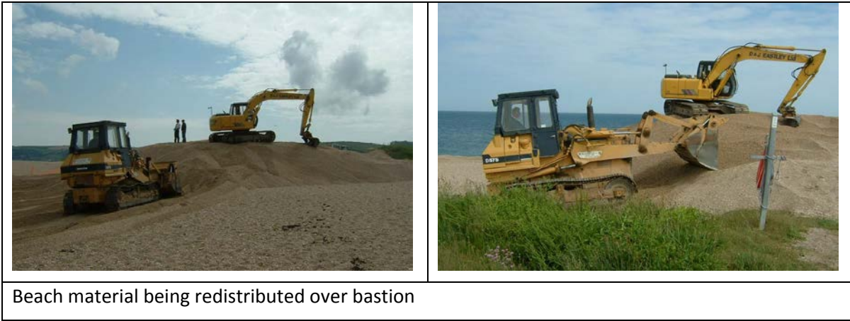
Figure 2.5 2005 bastion construction
