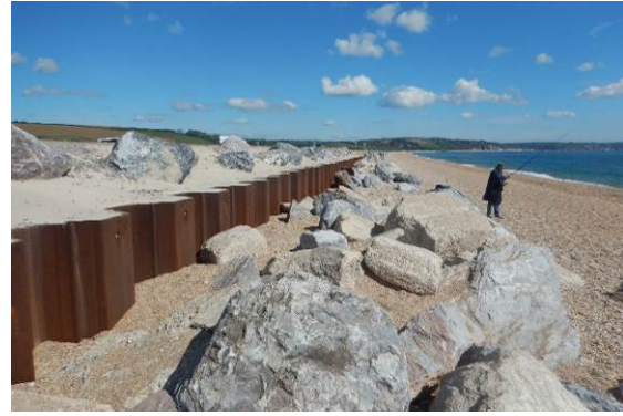
Extend of rock armour fronting the piled wall
