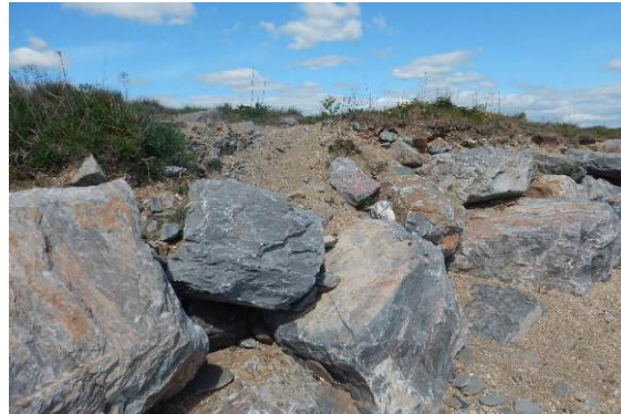
Erosion of the embankment behind the rocks
